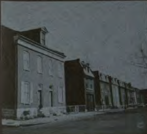
Beginning results of rehabilitation
